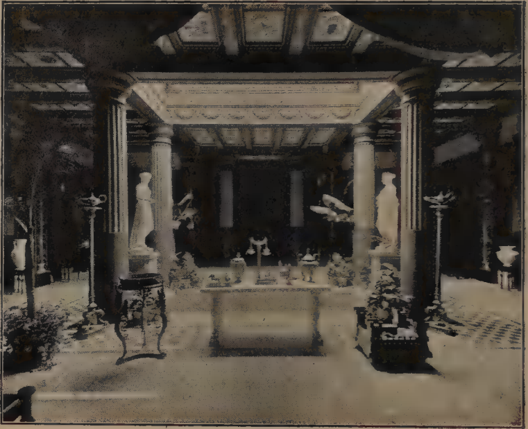
ATRIUM OF THE POMPEIIAN HOUSE AT SARATOGA SPRINGS, N. Y. Franklin W. Smith, architect.
